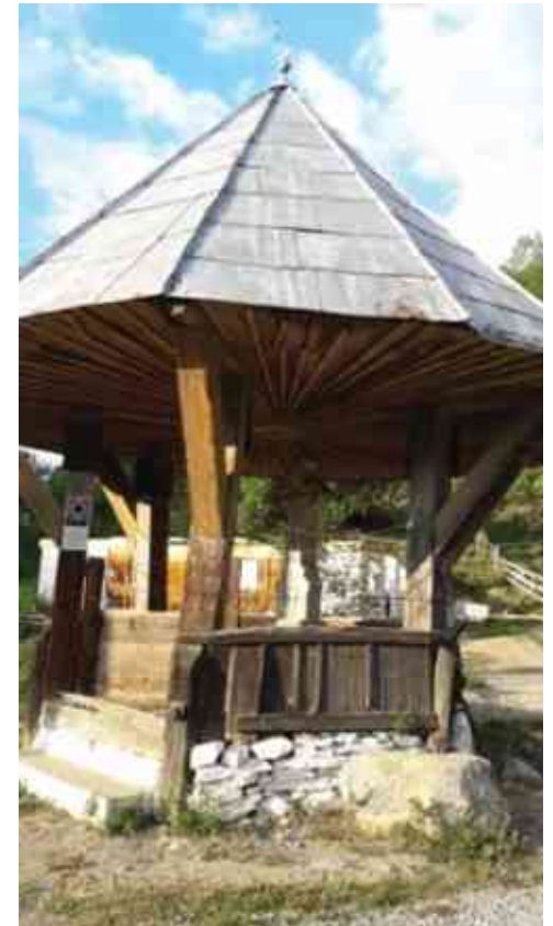
Fig. 1. The Cross erected by the Metropolitan Andrei Şaguna – 1897, on the site of a former wooden cross from 1847, and its protection structure in wood (photo credits: Elena-Codina Duşoiu, 2015).
