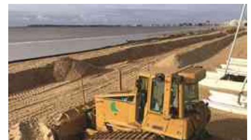
Fig. 4. Work for the creation of the Ecoplage, on the beach of La Baule, January 2019.
