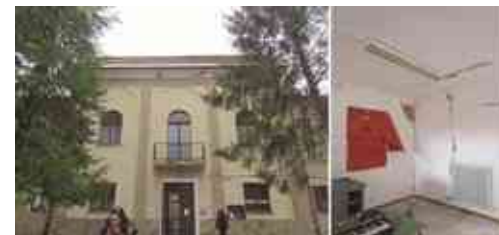
Fig. 4. Gualdo, the old school "Romolo Murri" after the earthquake: the main façade and a classroom (photo credits: R. Marmori, 16/12/2016).
