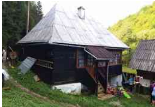
Fig. 6. The house of a shingle master on the Valley of the Abruzel river (photo credits: Elena-Codina Dușoiu, 2019).
